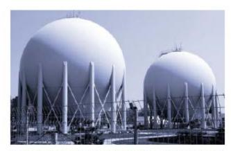
Spherical tanks are often used to store oil and gas at refineries, since this shape is the most economical to build.
