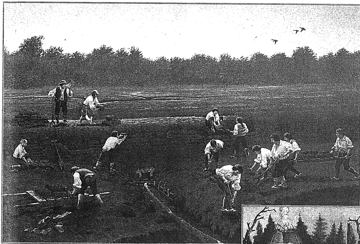
Above: Repairing a Dyke. The Acadians reclaimed low, marshy lands from the sea. Dykes were built of earth covered with sod. The dykes held back the water so the fields could be dried out and used for farming.
