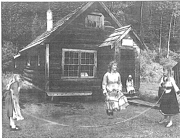
Figure 6-19 The old schoolhouse, which accommodated thirteen students
