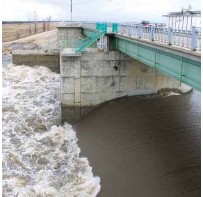
Floodway inlet control structure south of Winnipeg
