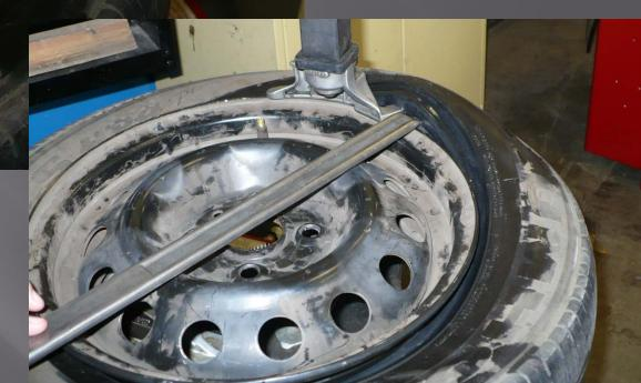
**Re-Set** Tire Tool o <u>Lift</u> ower Bead, Up on/the re to Assist.
